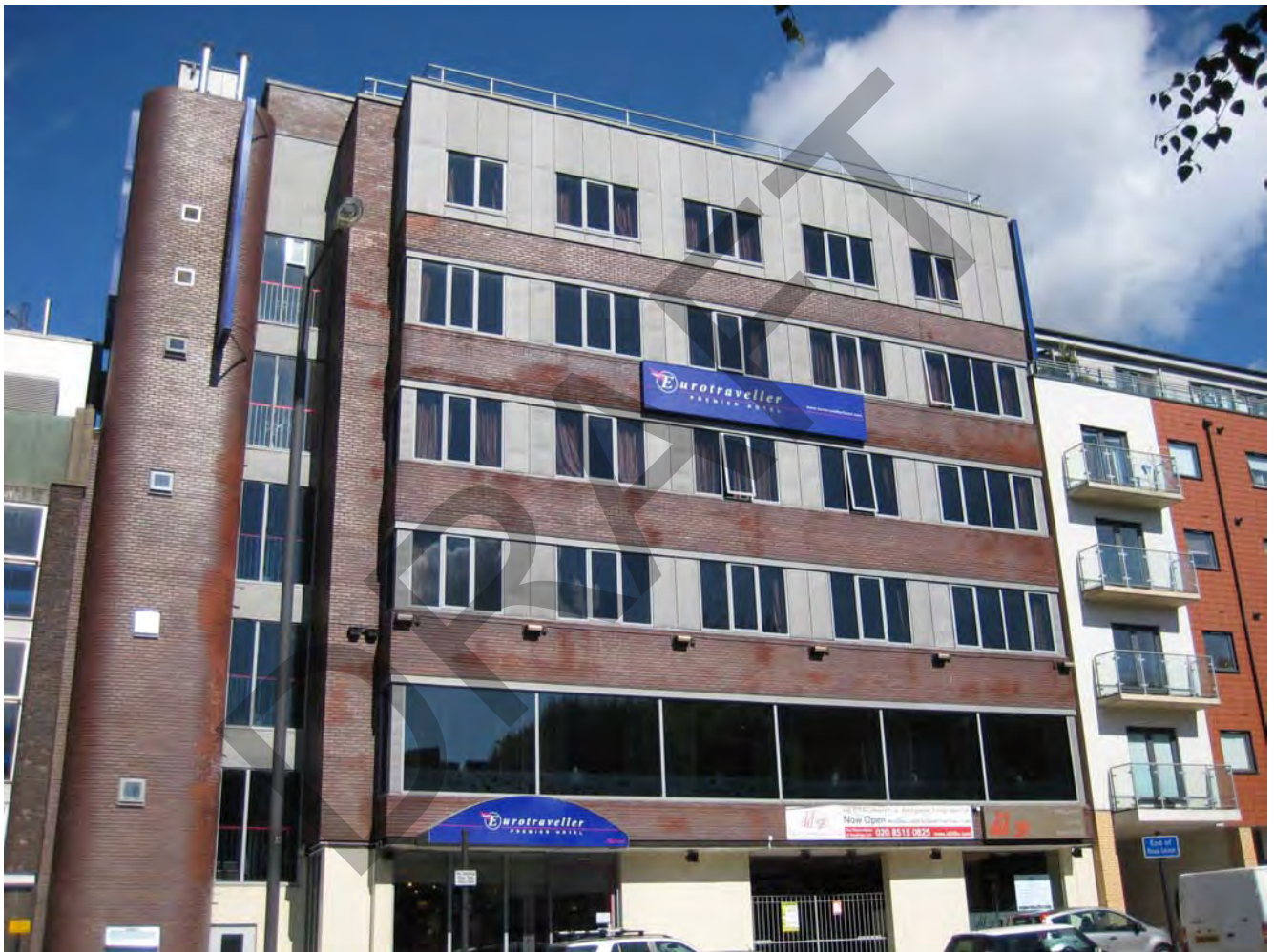
Picture 9 Scanmoor House
